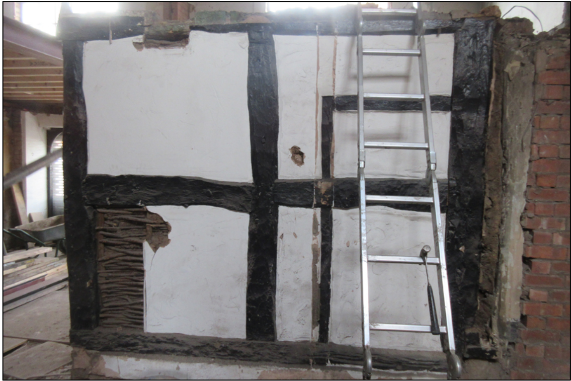
Figure 28: The timber-framed wall in No 10 OMP looking west, before removal, October 2019.
