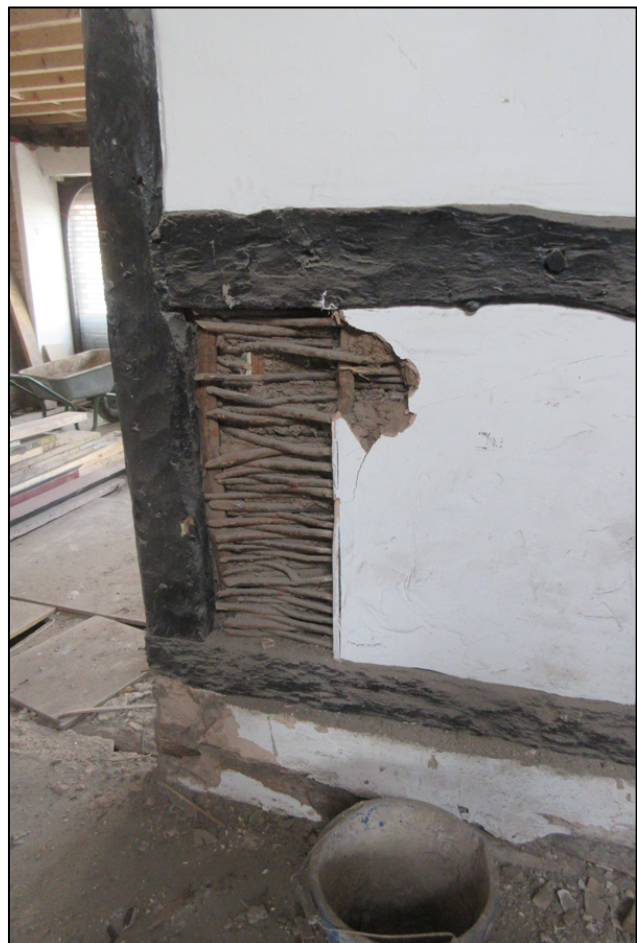
Figure 28: The timber-framed wall in No 10 OMP looking west, before removal, October 2019.
