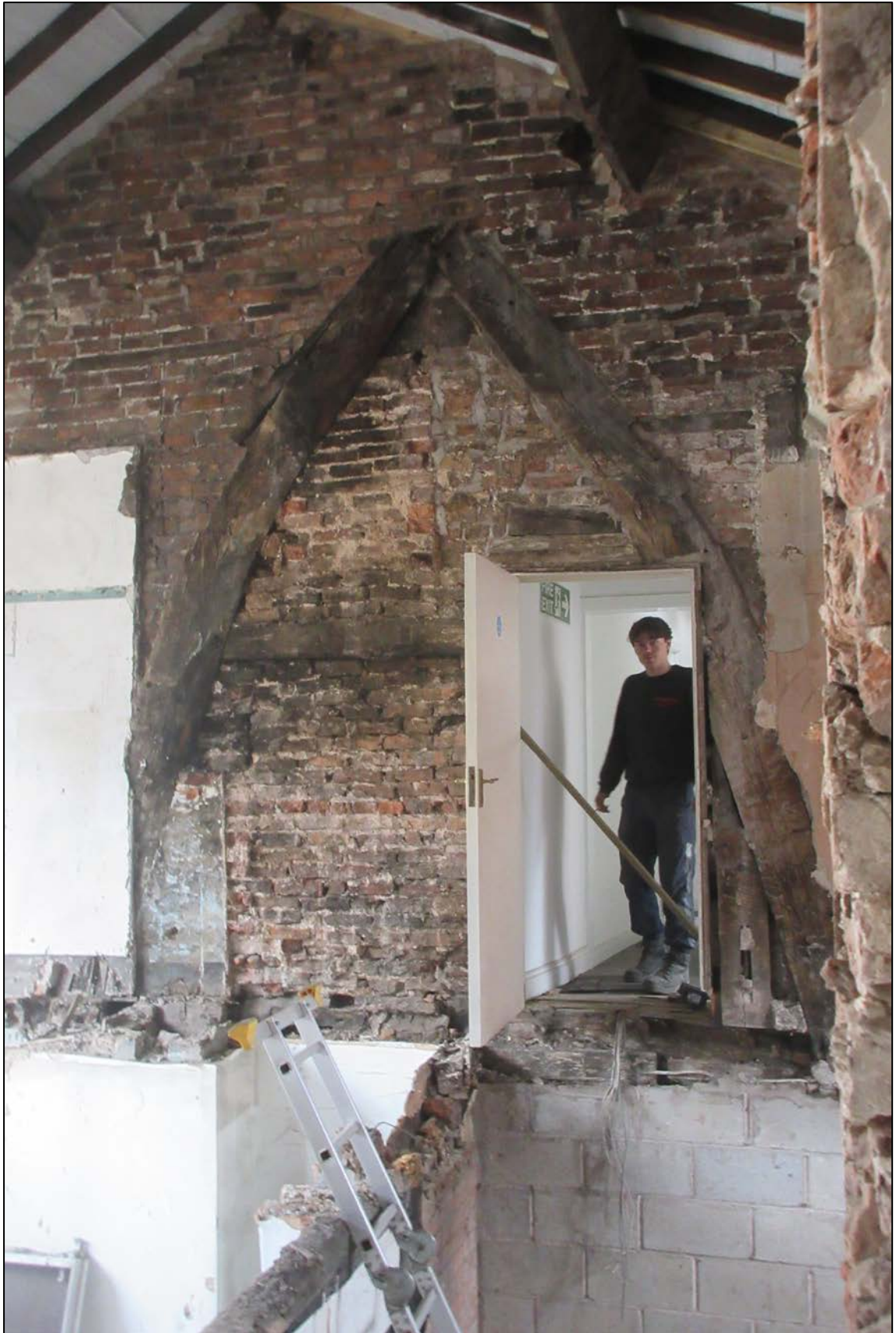
Figure 22: Cruck truss looking north with the timber-framed wall still in situ at the base of photograph.
